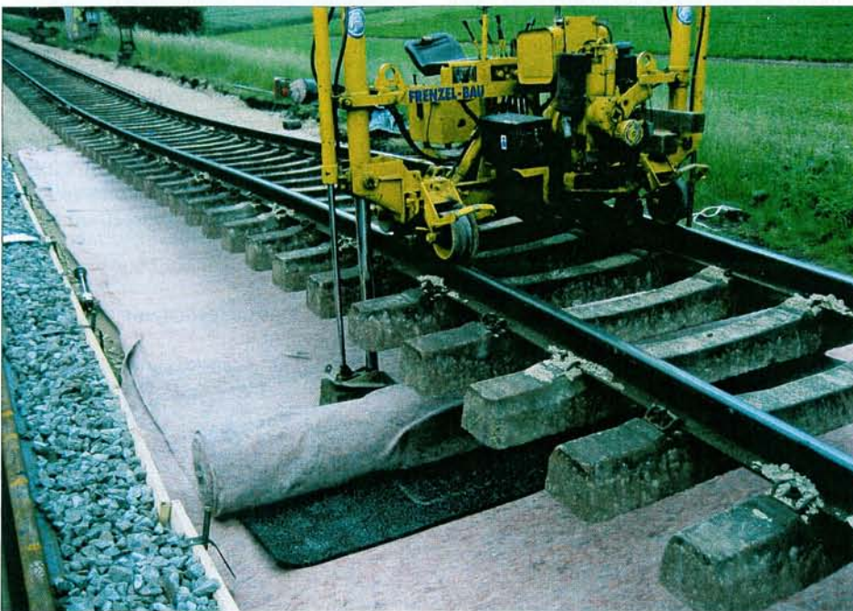
Fig. 3: Insertion of the drainage mats
