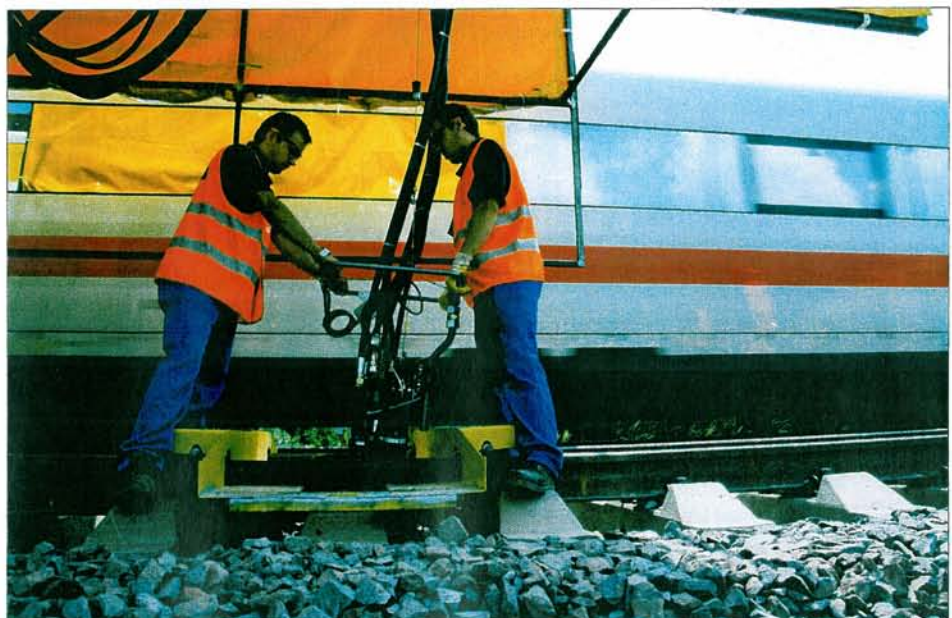
Fig. 1: High-pressure applicator machine applying raw material
